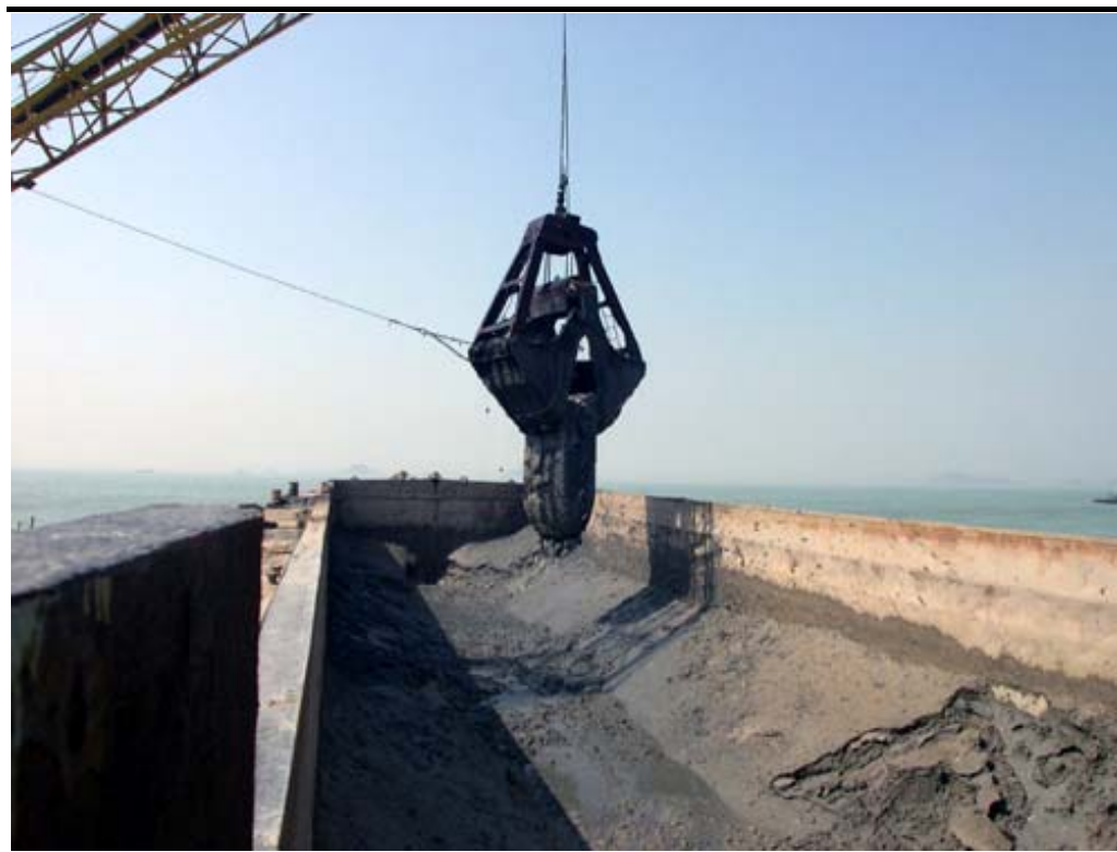
Figure 3.7 Dredge Bucket Dropping Sediment into the Barge
